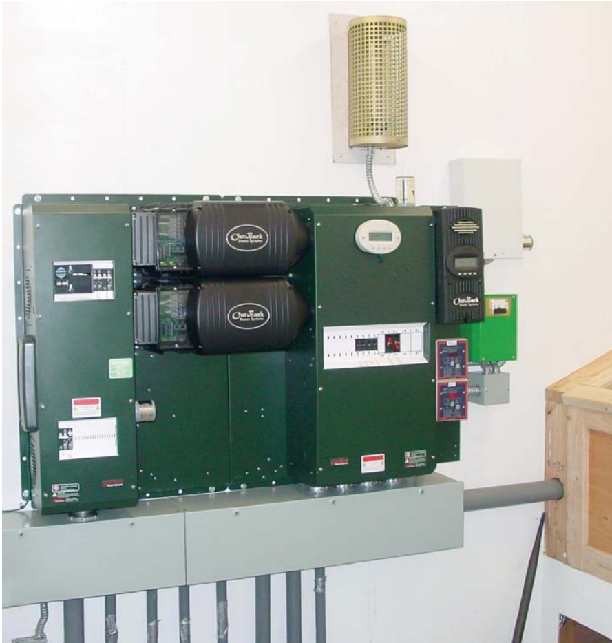
An OutBack charge controller and inverters are housed in the power shed, which is also home to a dump load, weather monitoring equipment, and the battery bank.
