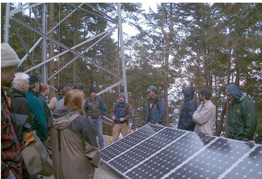
Kelly Keilwitz and E. H. Roy give SEI students instructions on the procedure for lifting the first array for placement on the tower.
